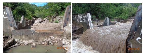
Figure 3-2: La Simona v-notch weir repair on 12 October 2016 and subsequent flood event on the 18 October 2016
