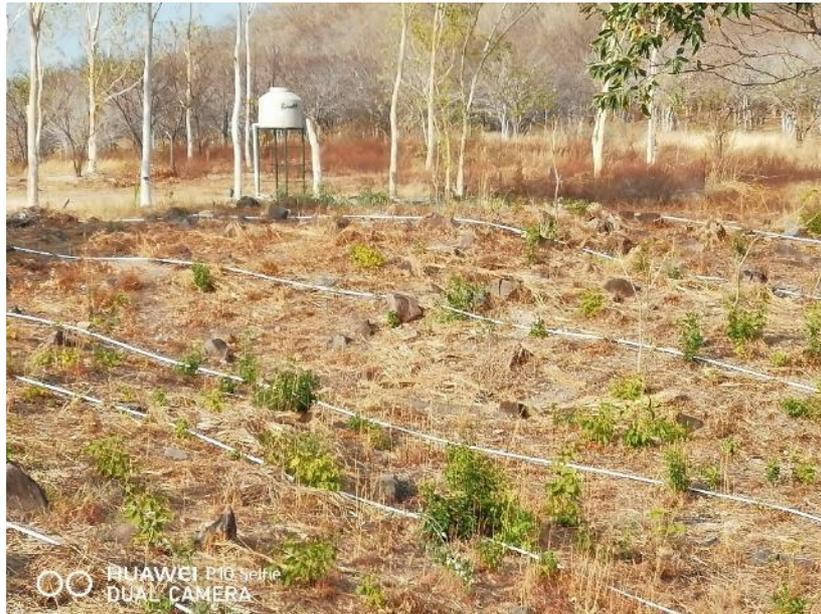
*Photograph 3.2.3.1.a Drip irrigation system installed in ALPHA 6 reforestation area*
