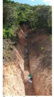
Trench sampling on the America Vein to test for gold mineralisation in the wallrock of the historic mine workings.
