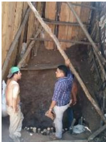
Illustration 14: As part of the inspections carried out, depth of workings and type of support are evaluated at the worksite
